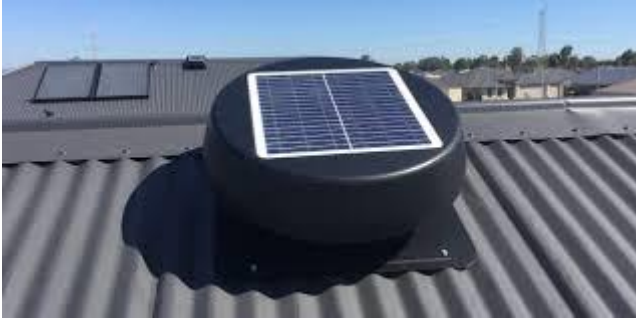
Photo 1 Solar power ventilation
