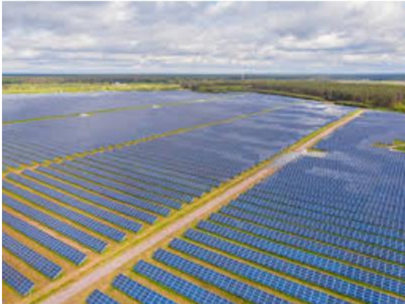
Figure 2. Large-Scale Utility-Scale Solar Energy Project
